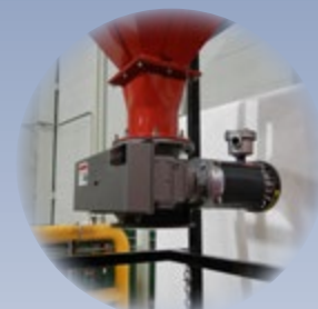
Rotary Air Locks for continuous discharge
