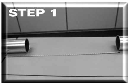
Measure distance to be spanned.
