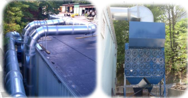
Dust Collection & Heavy-Duty Ducting Installed on Transportation Equipment Blast Room
