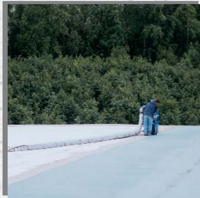
Steel storage tanks
