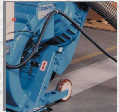
Concrete warehouse floors
